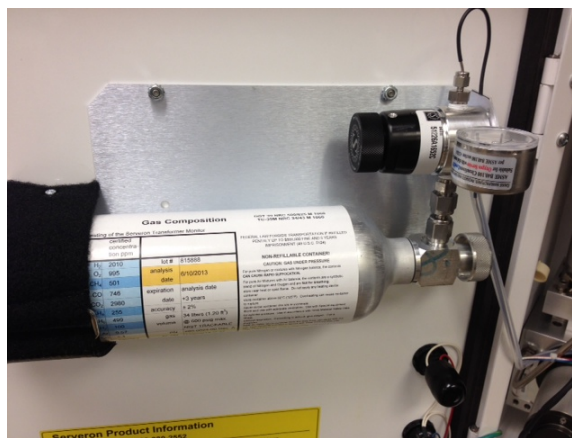
Figure 18: Installed Verification Cylinder
